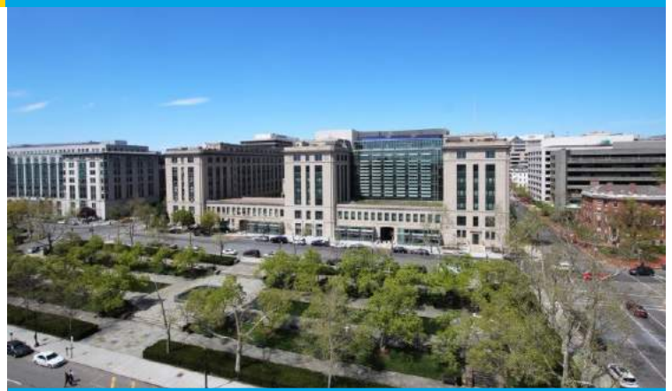
Prototypes were tested at the General Services Administration (GSA) Headquarters in Washington D.C. (Photo from GSA)
